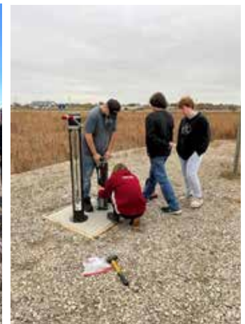
Installing the Repair Stand
